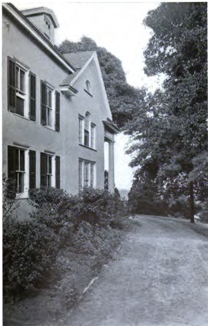
THE SIDE OF THE HOUSE, AS IT NOW APPEARS
